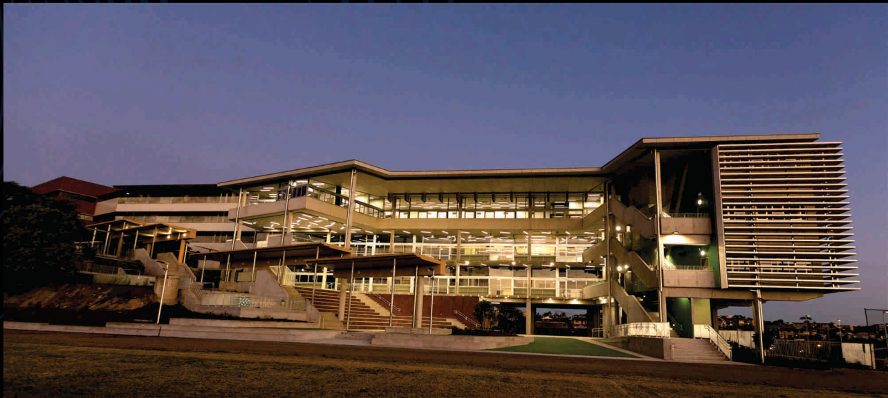
VILLANOVA LEARNING CENTRE PROJECT COST $1.36M (Electrical)
